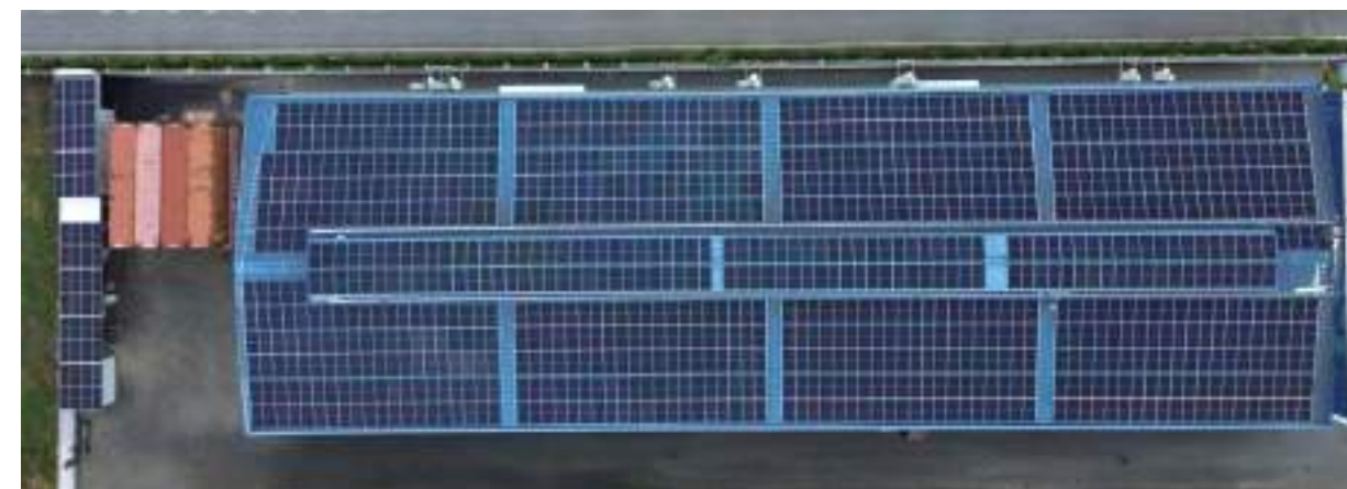
>> Factory Rooftop Photovoltaic Panels
